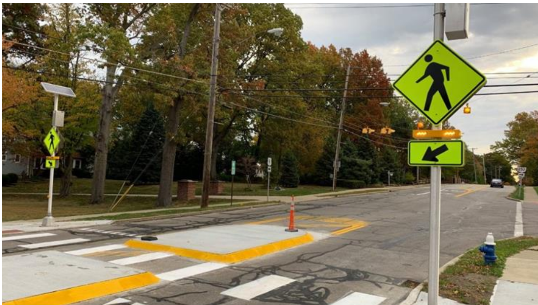
Figure 8: Raised medians create vehicle lane pinch-points, which can double as a pedestrian refuge island. Crosswalks can be further enhanced with flashing beacons.
